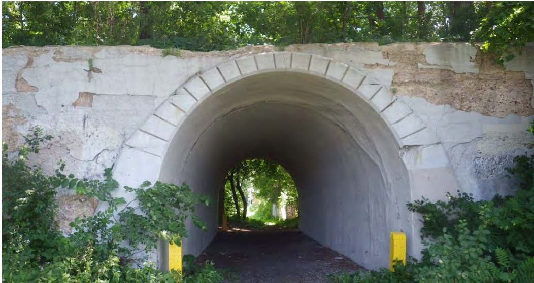
Figure 91. 14-foot-wide concrete arch bridge near Clarence Court (MnDOT Bridge R0438, RA-SPC-11140, contributing). This structure carried the StP&D railroad roadway (currently the Bruce Vento Trail) and allowed local traffic to pass under it. It may have been installed when the 1887-1889 trestle was filled in 1908. 128
