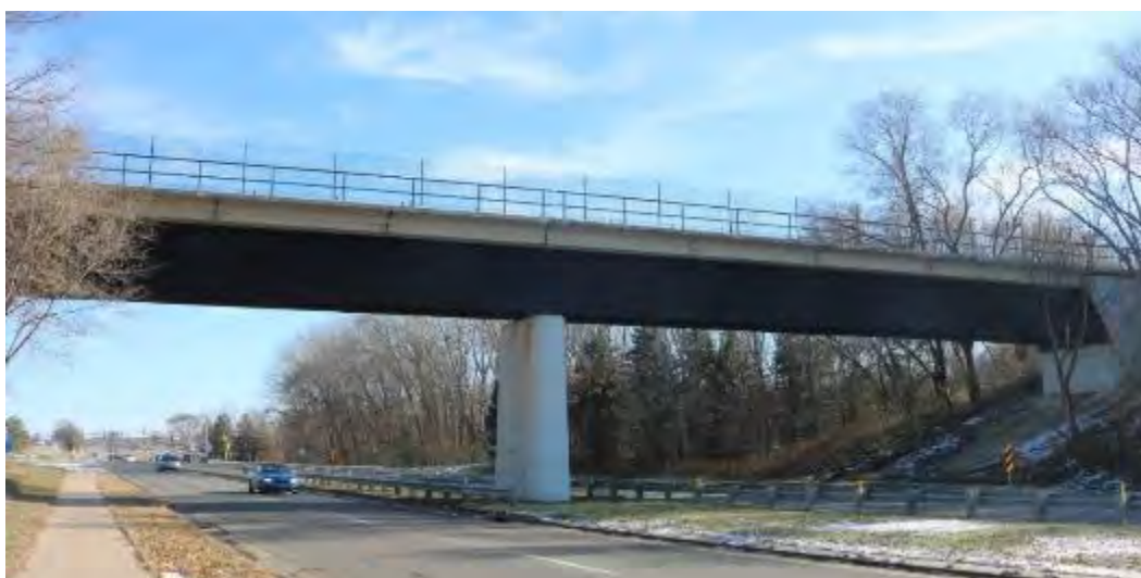
Figure 47. Bridge 62529, view facing east along Beam Avenue, showing the 25-foot vertical clearance that is consistent with the height of the original LS&M railroad roadbed at this location.
